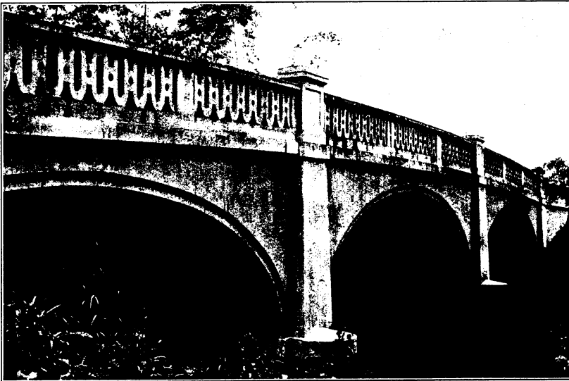
Fig. 2. The bamboo bridge replaced by a modern concrete structure in which Rizal cement was used. This is one of three such bridges in the same locality.
